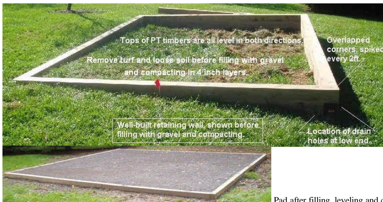
Pad after filling, leveling and compaction.
