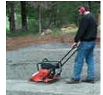
Using a plate compactor to pack the gravel
